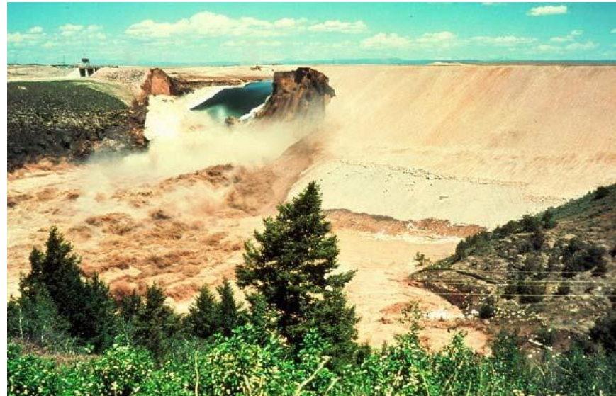
Williamson Mine, Tanzania , 7 November 2022 , Dam wall breach
